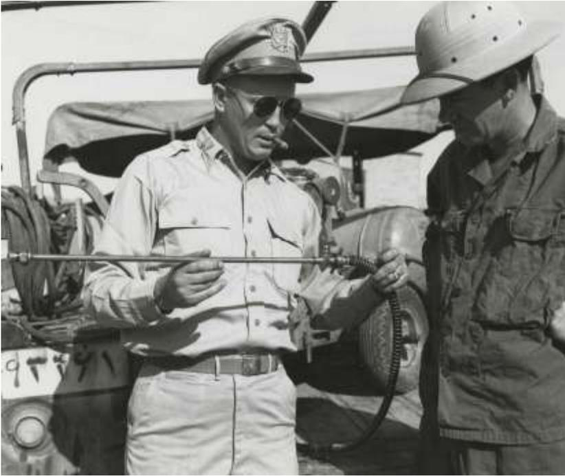
DDT was an enormous help against insects and insect-borne diseases in WWII. Here, two soldiers examine an adapted compressed-air paint sprayer used to propel a kerosene/DDT mix.
